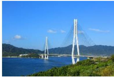
Anti-corrosive coatings (Stricter environmental regulations)
