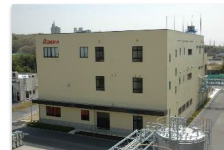
▲ Mie Plant's manufacturing building
