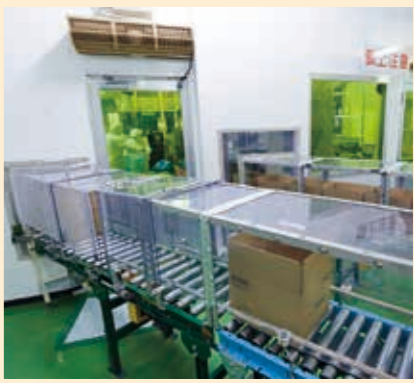
Installing tunnel-style covers over cardboard box conveyor lines
